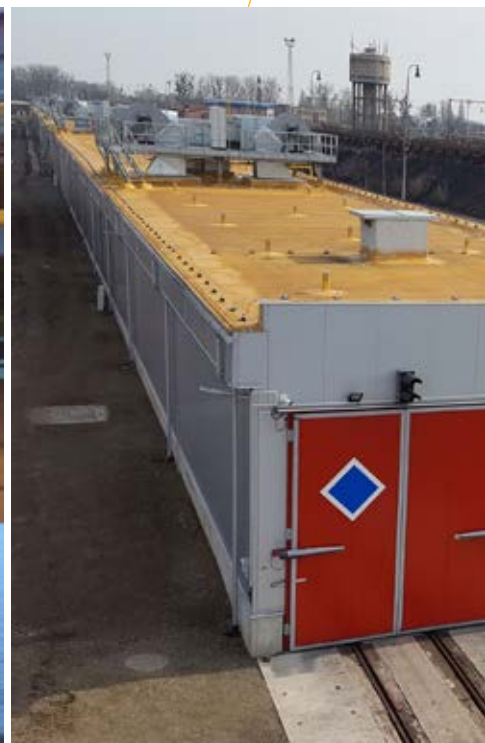
II. Rozmrazovacia hala. 2nd Defrosting Hall.
